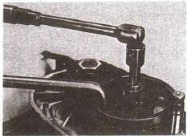
25. Holding The Clutchbody With Special Holding Tool
